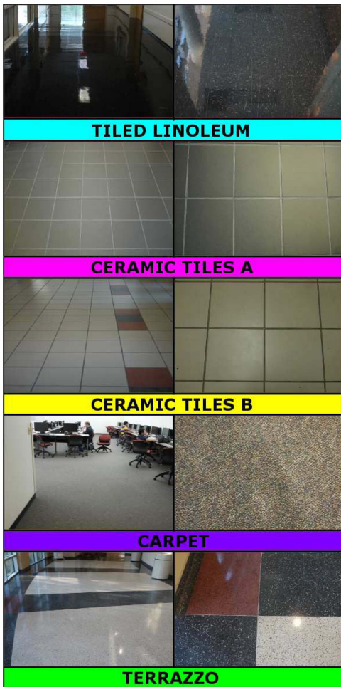
Fig. 5: Five types of terrain found in the ECSC at UTD. The left column has pictures taken from a distance, while the right column shows close up views of each type of terrain.
